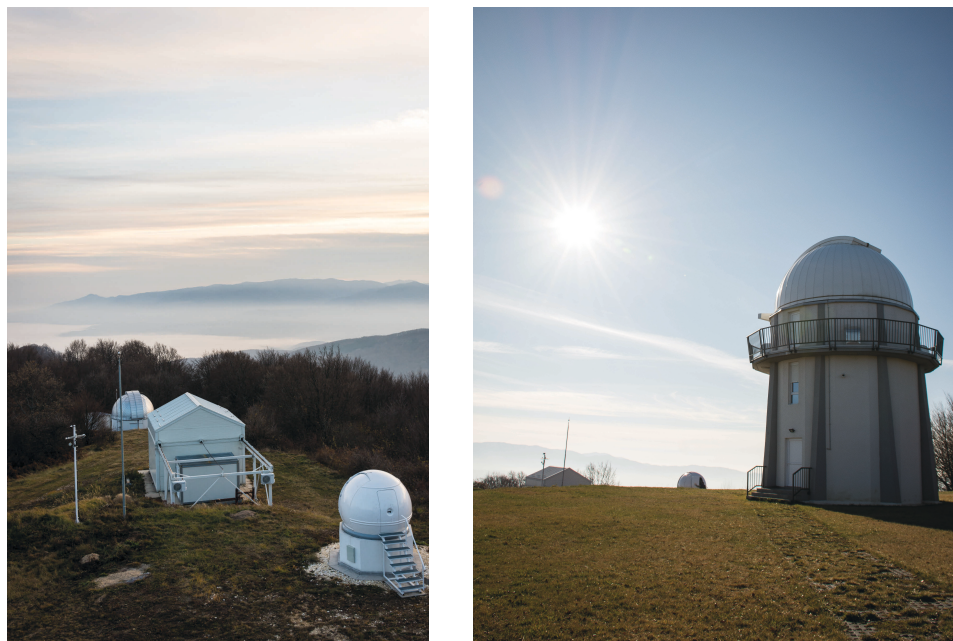
Figure 6: Pavilions wherein ASV telescopes are situated: left panel photograph - from left to right: pavilion with 6 m dome, pavilion with movable roof, pavilion with 3 m dome; right panel photograph - pavilion with 7 m dome where is 1.4 m telescope.
