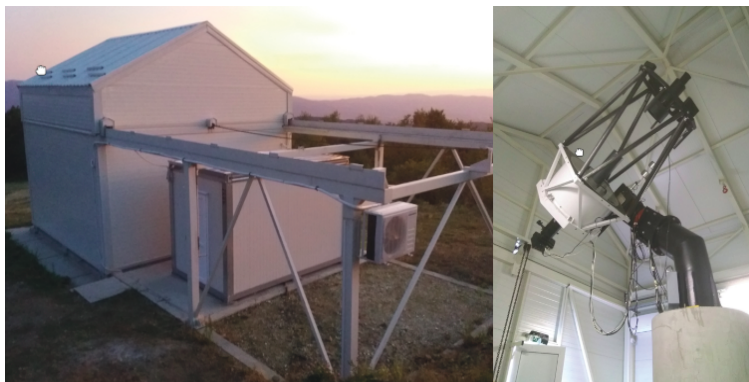
Figure 2: Left, the roll-roof pavilion designed to temporarily house a 140cm "Milanković" telescope. Right, the 60cm 'Nedeljković' telescope, which is currently in this pavilion.
